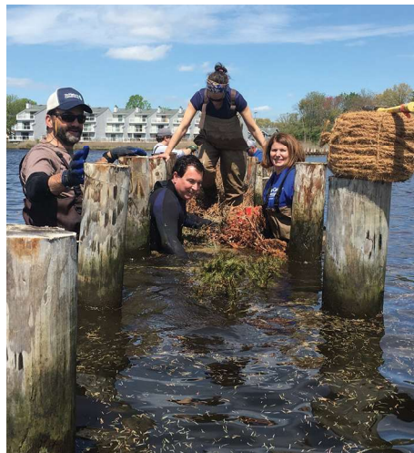
Volunteers carefully place and secure Christmas trees to branch boxes. © Princeton Hydro
