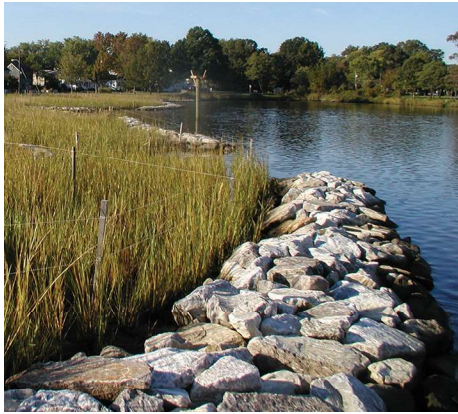
Example of a marsh sill from a site in the Chesapeake Bay Estuary. © Chesapeake Bay Trust.
