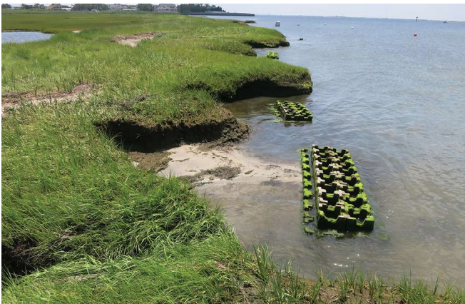
Geotube sills (top): Installed in 2010, two heavy-duty polypropylene tubes filled with fine sand were installed parallel to the shoreline to intercept oncoming waves. Oyster Castle® Breakwater (center): Units were assembled in a larger pod to form a breakwater a few units were seeded with oyster spat to jump-start shellfish settlement (Mordecai Land Trust). Marsh sills (bottom): Oyster Castles® were assembled in smaller pods along the marsh edge to stem erosion, trap sediment, and encourage plant growth (Mordecai Land Trust).
